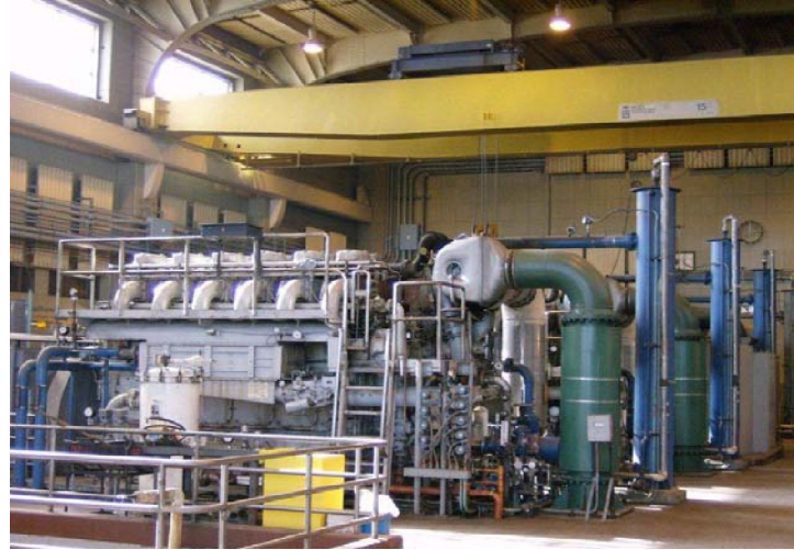
CHP system at Coney Island WRRF, NYC
