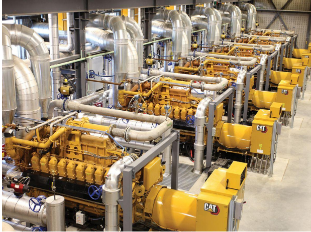
CHP system at landfill, Quebec
