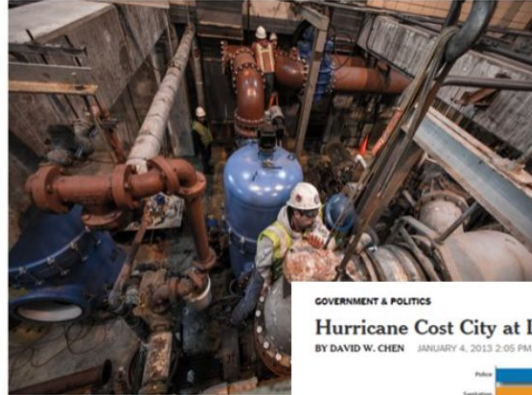
Workers this week replacing pumps at the Bay Park sewage-t
